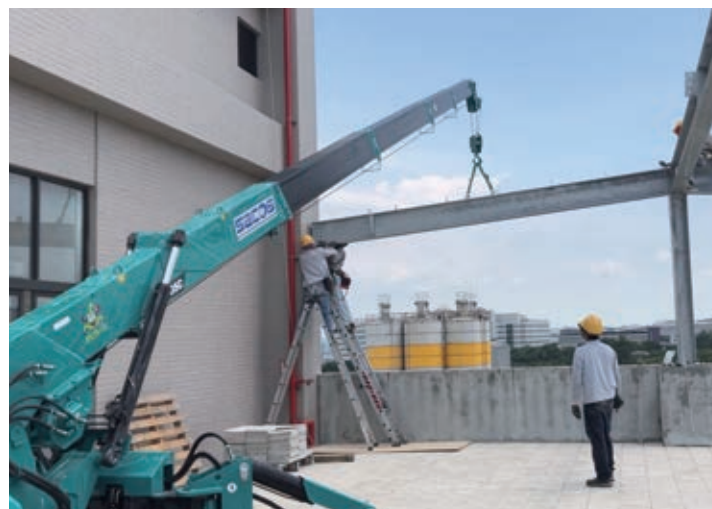
MC305C Solar Frame Erection
