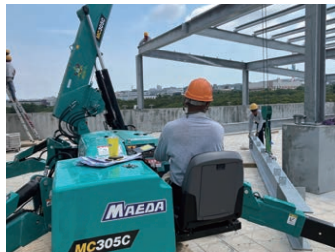
MC305C Solar Frame Erection
